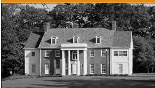
Limited housing is available in the gracious Hospitality House on the CTS campus.
